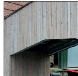
Wood sealer four years after installation
