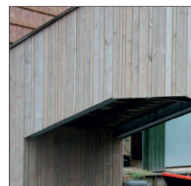
Wood sealer four years after installation
