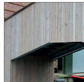
Wood sealer four years after installation
