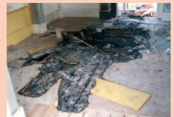
Graham Price, the Council's Head of Property Services said: "The main part of the structure was still intact, mainly because of the DRICON fire retardant treated timber used in its construction. If this material had not been used, the entire pagoda, with construction costs of over £250,000, would have been destroyed.
